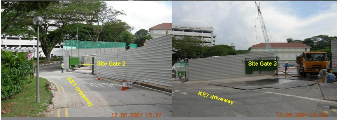
Traffic control at junction of College Road and KE7 Drive
