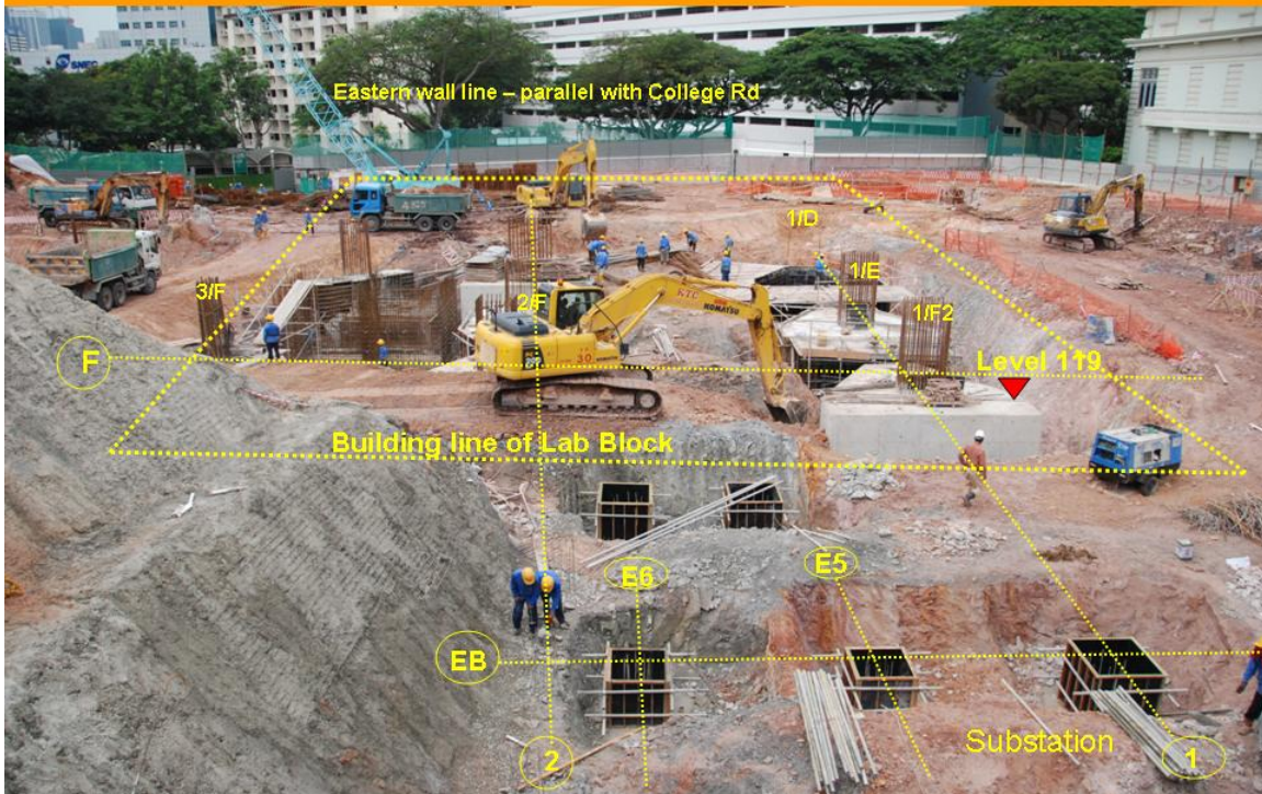
25 June 2007 - Lab Block & Substation pile caps under construction
