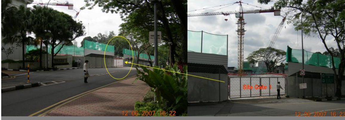
Site fronting College Road
