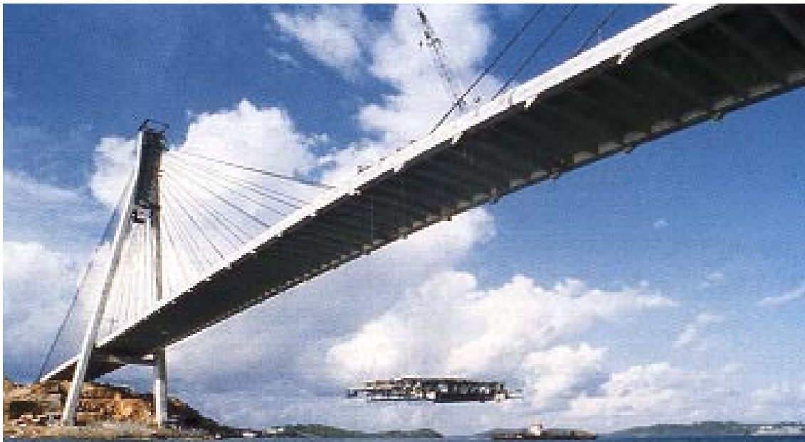
The photograph shows one of the last construction stages.
