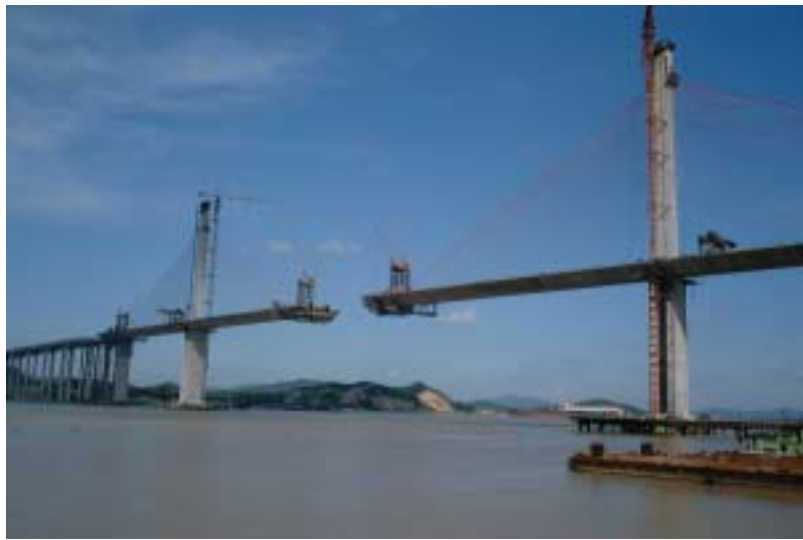
Fig.2 The Yamen Bridge during erection
